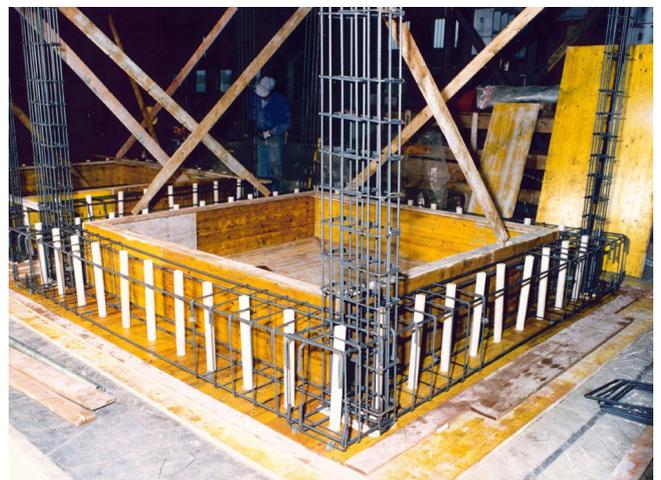
Fig. 4. Detail of the reinforcement.
